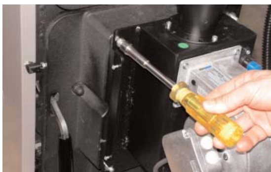
Fig. 13.11: Assembly of burner
