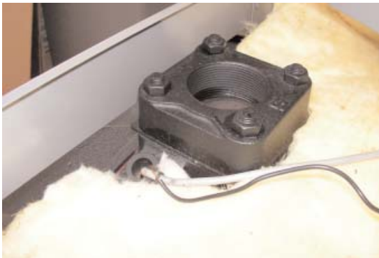
Fig. 13.16: Insertion of the probes into the sheath
