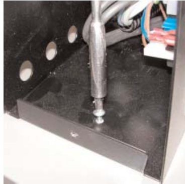
Fig. 13.14: Fixing of control panel
