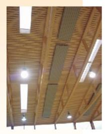
The distribution pipes normally extend high up, nearly at the level of the roof. Installing them requires the use of scaffolding or elevator platforms.
